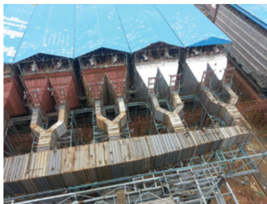
Glandular Guillotine Isolators for ESP Inlet/ Outlet at 2x660 MW Jaypee Negri Power Plant
