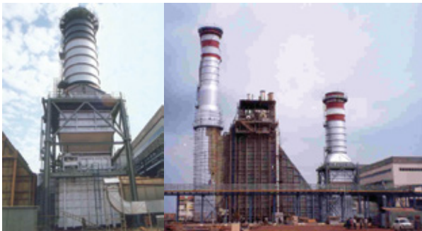
Total GT Exhaust System executed by Fouress for Siemens V942 Turbine at BAPL, Samalkot 230MW CCGP through BSES, Noida
