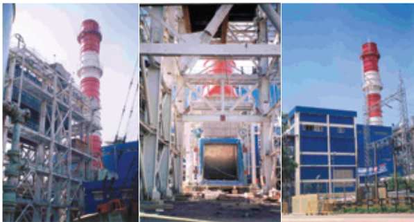
Total GT Exhaust System executed by Fouress for GE Frame 9E Gas Turbine at AES Kalinitissa, Sri Lanka (168 MW CCGP) through L&T, Mumbai
